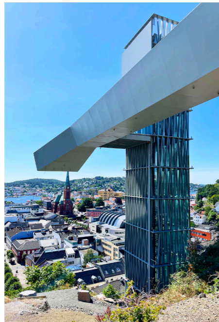
Freestanding elevator (Arendal)
