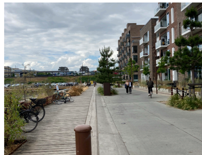
Road structure, Nordhavn (DK)
