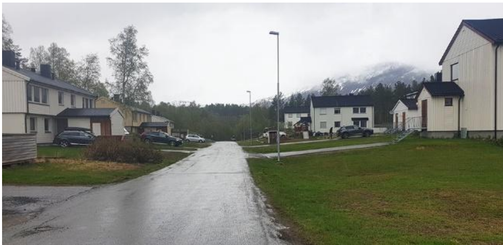
Figur 15: Boliger i to rekker langs Toftakerlia -veien. (Foto: 3RW, befaring 2023)
